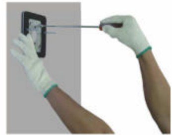
1. Level bracket and install on wall.
